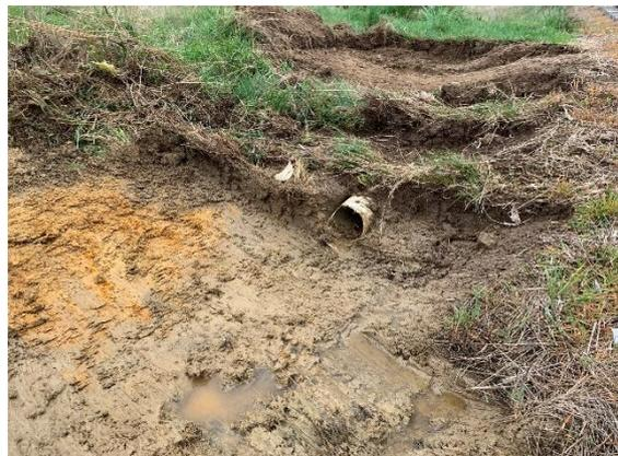
*Work on the cess uncovered buried pipes which when cleared made a big difference*
