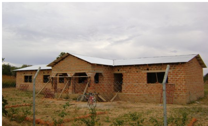
House under construction
