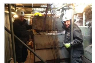
The chimney was found to be in good enough condition not to need any major work doing to it. It awaits a capping stone, placed on smaller blocks of allow stone. to ventilation to the chimneys shafts. It will look particularly handsome when it is finished and repointed, as will the whole building.
