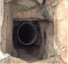
Next to the old chimney is the second flue, which has obviously been built and lined at a different stage in its history. It serves the same purpose and will enable there to be some
