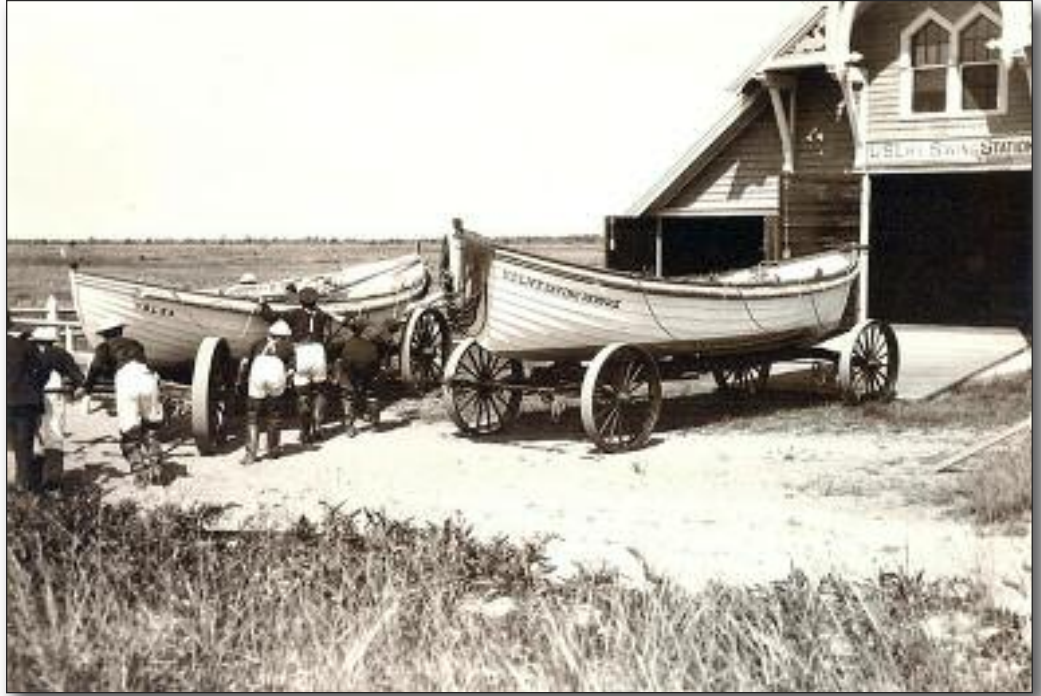
Galveston USLSS Station probably looked similar to this before the storm. (U.S. Coast Guard Photo)
