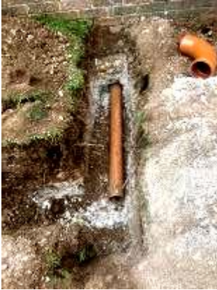
(top right): pipes from dummy drain and real soakaway combined and sent to the right under the wall
