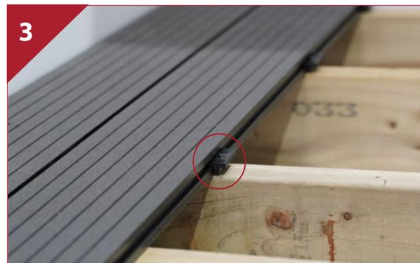
Push the second row of boards into the previous installed row of boards making sure that the deck board grooves are in tight on the clips. Continue to keep inserting clips and boards in this way (using one locking clip per board).
