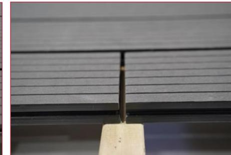
Board ends butted together must be supported by separate joists and have a min 5mm gap for expansion. Failure to do this may result in structural failure, swelling and warping. There should be a spacing gap left between the double joists to allow rainwater/debris to fall through the boards.
