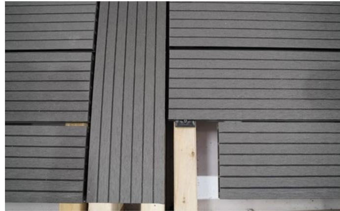
**Note: Gap for water to run off board ends to the ground.**
