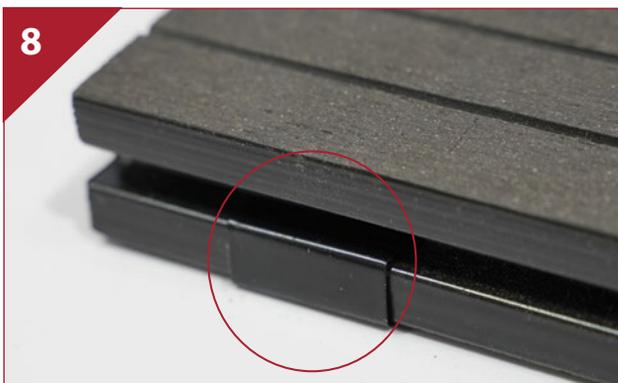
For the last row of boards use a start/end clip in line with each joist. You need to use these clips even if you putting on a fascia board. If you can not slide in the board, the boards can be fixed with screw at 45 degree angle.
