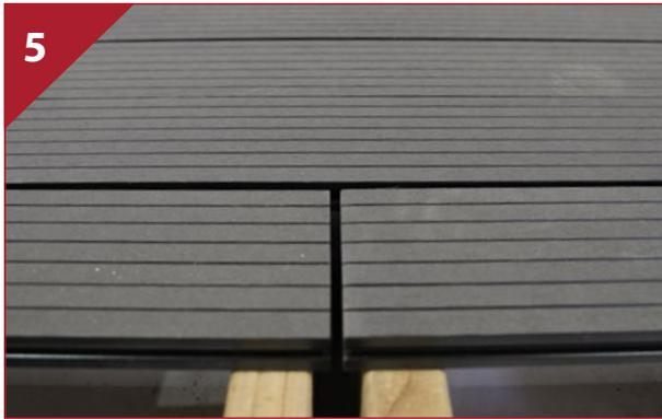
When butt jointing boards along the length of the deck you must leave a 5mm gap for seasonal expansion and contraction - see diagram above. Note comments on point 6 regarding double joisting. Boards must not meet across one single joist and must be sealed to prevent swelling, cupping and splitting.
