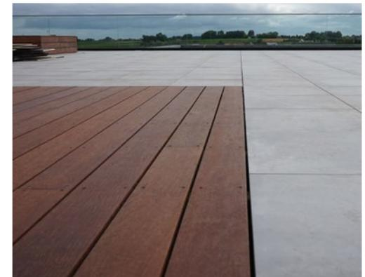
Pedestals give great flexibility for installations and make it easy to allow decking and paving to be installed easily in the same area.
