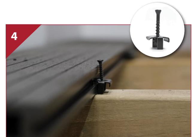
It is very important to install one locking clip per board onto the joist nearest the centre of the board. This helps maintain a consistent expansion gap at the short end. Failure to use the locking clip will result in uneven gapping at short ends. **Attn: Each board only requires one locking clip in the middle. The teeth should always face the same direction.**
