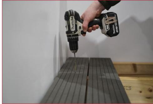
Composite decking should only be installed using correct clips and fixings. Failure to do this will affect the structure of the deck as well as warranty. Never screw directly through the boards. Steel joists >2mm must be pre drilled and specific Steel Joist Installation Kits must be used.
