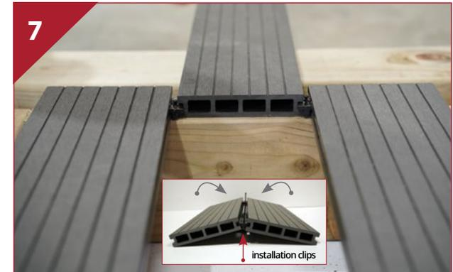
If not framed by wall or building on each side, the second last row of boards can be slid into position after you have fixed the last row and the clips for the second last row have been fixed into position.
