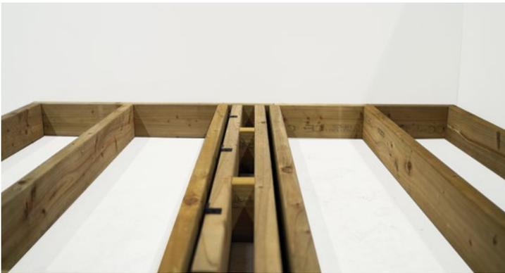
**Important:** All Ultrashield board ends meeting the breaker board or at deck end should be sealed with a water based polyurethane matt exterior varnish to prevent moisture penetrating the board core. The boards should be predrilled with a 3mm drill bit before screws are fixed at 45 degree angle to fix the breaker board. Its important to predrill before screwing as this prevents the boards cracking later. A starter clip can be used on one side of breaker boards.
