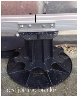
Joist joining bracket
