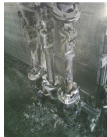
Fig.7: [REDACTED] bus bar system during the installation in 2007, during the fire and after the fire
