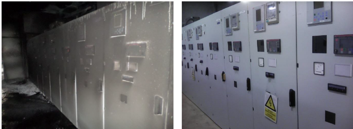
Fig.8: Centrale 4 switchgear before and after cleaning
