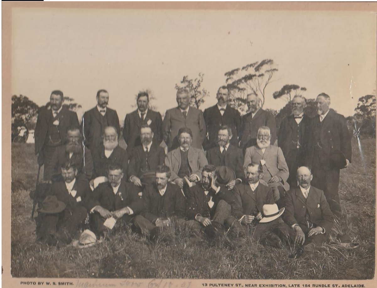
Photograph courtesy of V Connell, Mypolonga, 1974. MLHC 121.
