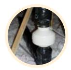
The radon fan is located in an unconditioned space, so radon does not enter the home if the fan or pipe above it leaked. The fan is plugged into an electrical junction box or hard wired with a switch.
