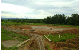
Fishpond construction finished.
