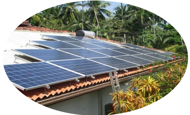
5 Kwp Roof-top installation – Martinique FWI
