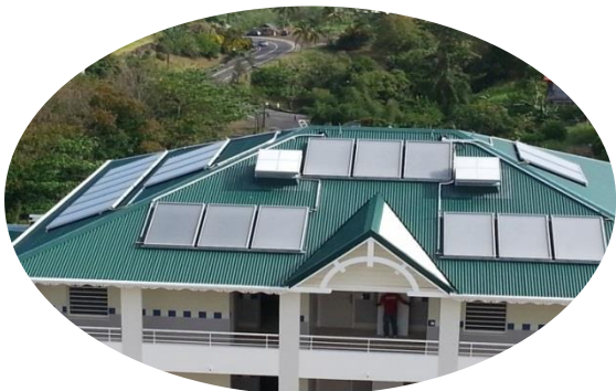
Collective Solar Water Heating Installation - Martinique
