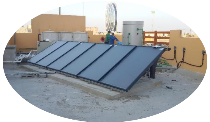
Collective Solar Hot Water Installation in Abu Dhabi – UAE
