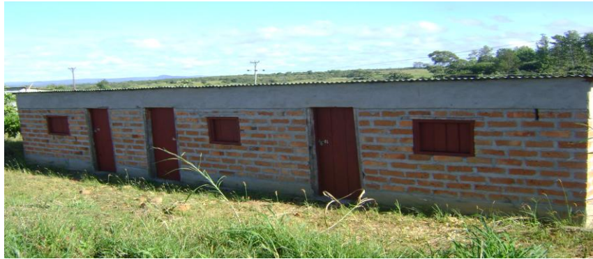
Chicken run building finished
