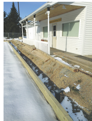
installation of new plinth
