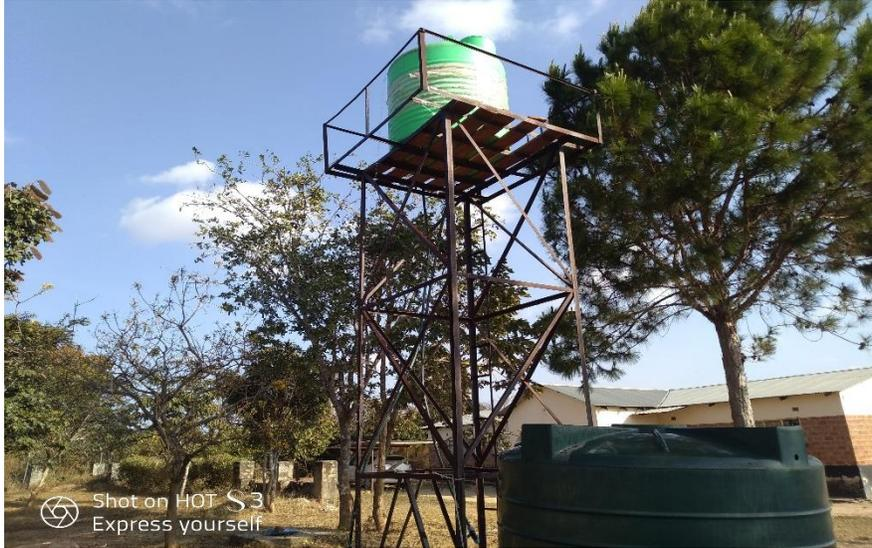
**The overhead tank has been also mounted and water is connected.**
