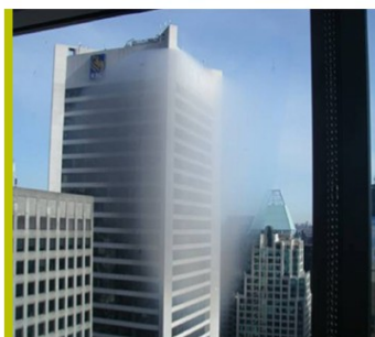
Volatile fogging occurring during periods of warm weather in direct sunlight
