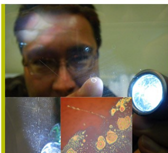
Examining hazing that could not be cleaned (Corrosion of silver low-e coating inside IGU)
