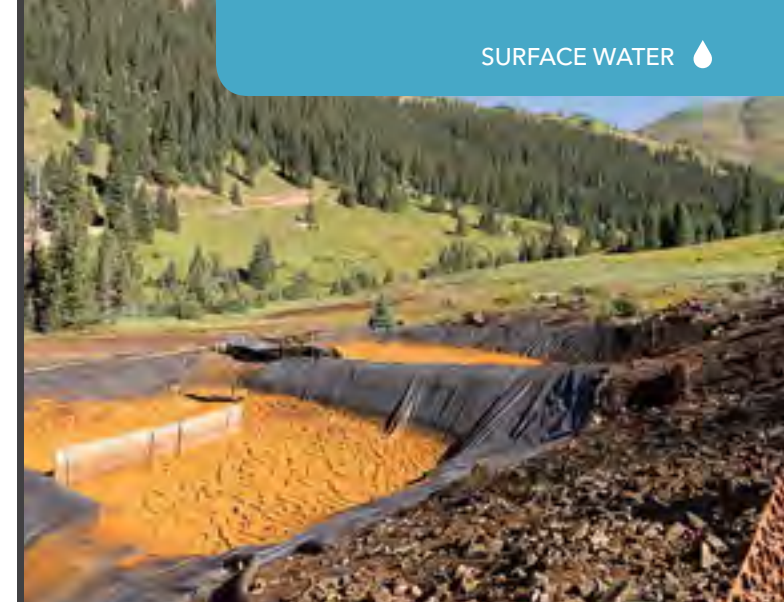
Above: Treatment ponds close to the Gold King Mine Below: Water Monitoring in the Animas River with a YSI handheld multiparameter meter.
