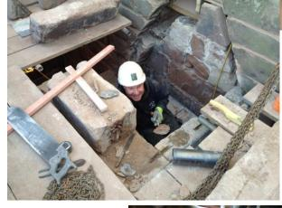
Shown here, each stone being glued into place with the use of stainless steel dowels, which are dropped between each stone. Paul is an expert at this job and takes delight in his work!
