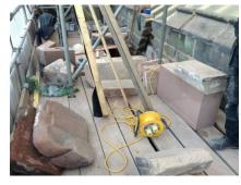
The stone roof above the Oratory is now half complete, but what seem to be stone slates are in fact huge blocks of sandstone, now firmly in place with a sealed lining between each block.
