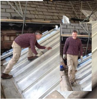
Matt the roofer is very pleased with progress so far, although he would much prefer working with lead, which he has done since he first started work. Sadly we cannot risk roofing with lead at a low level anymore, owing to the risk of theft.
