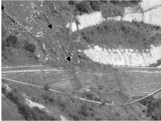
Fig. 5 Detail: road after landslide.
