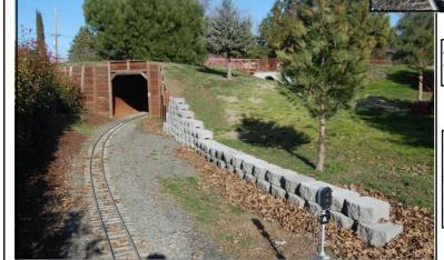
Left: one of the new cement brick landscape walls Elvin has constructed to assist in strengthening the soil over tunnel #2. Elvin will also construct a wall next to tunnel #3 along the small access road between the two tunnel portals.
