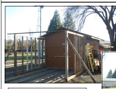
As of March 3, 2013 the 10 foot extension to car barn #2 has been framed in and the stringers will be added for the roof in a few days if the weather holds out. The current doors and front will be moved to the front end of the new walls and a side door added to lock the "train doors" from the inside like in the engine house.
