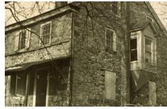
side of the Mansion was severely deteriorated as was the oriel window on the second floor on the south side. These windows were both removed. The concrete blocks, that are visible inside and stone on the outside were expertly installed. Today, looking at the Mansion, you would not know these windows are missing. As you can see we
