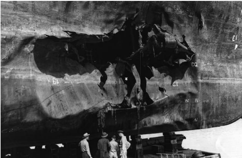
Damage done by a torpedo hit in the hull of the William Cullen Bryant . She was attacked on July 21, 1942, a little more than 40 miles from Key West. Miami News Collection, History Miami, 1989-011-18401.
