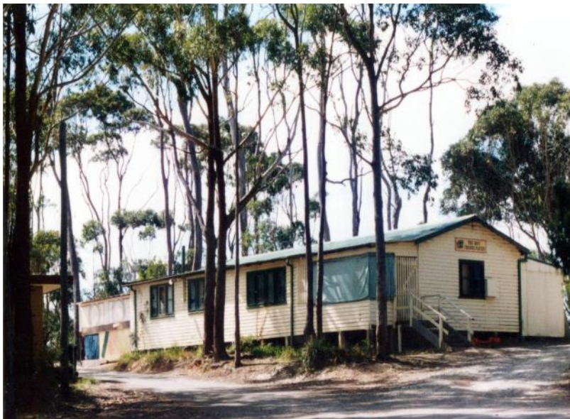
Batehaven Hall, Observation Point. Demolished. Memories?
