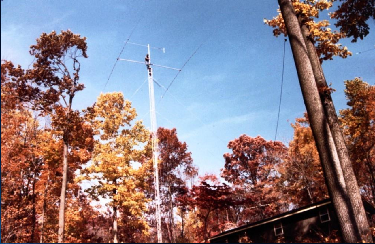
70' Rohn 25G fold-over tower KM1A (SK) Killingworth, CT
