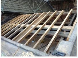
New roof spars made and fitted by the timber specialists Robinson's, begin to create the new roof over the Rectors Vestry, supported by the 17th century trusses and purlins
