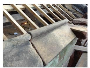
The restored roof is taking shape, soon to be covered with plywood. The pitch of previous roofs can be clearly seen
