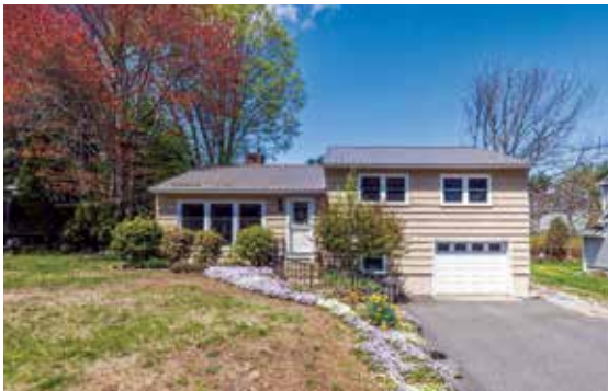
31 Edgewood Road, Wells
