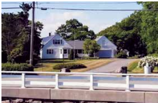
22 Pier Road, Kennebunkport
