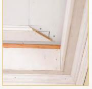
No blocking? No problem. When we need nailing in the center of a joist bay, we carefully cut a rectangle in the drywall, insert a slightly larger piece of plywood, and secure it with screws (center). Positioned every 2 ft. to 3 ft., these nailers provide enough support for the ceiling soffit and crown (above).
