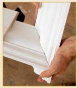
if butted. Yellow glue or urethane construction adhesive keeps the joints from moving later. The configuration shown is made from stock profiles available at any lumber-yard. The ceiling frieze, a baseboardlike flat applied to the ceiling, forms the base for the final piece of the puzzle, a 3½-in. crown.
