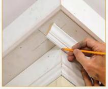
Marking accurate miters in place. Outside corners are never perfect, and rather than run back and forth to the saw, I hold one side of the miter in place and make a pencil line above and below where it intersects with the other half. After marking both halves, I transfer the marks to the molding, and using the laser guide on my saw (center), I cut the miters.
