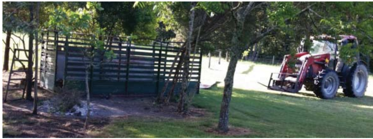
Cleared site with the Cattle Crate moved in to place
