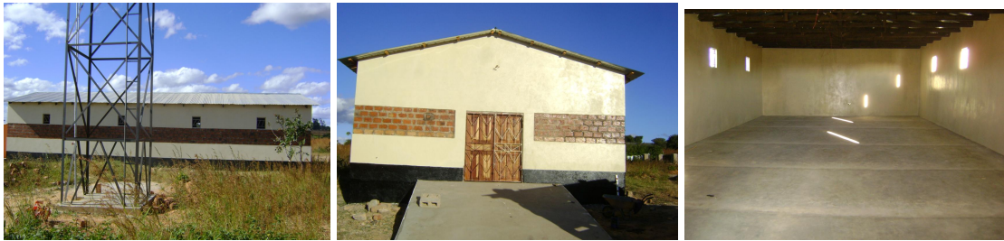
Storage shed side, front and inside view.
