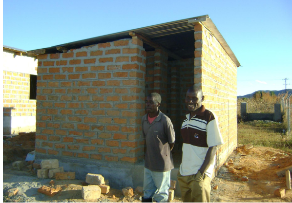
Four doors VIP Toilet
