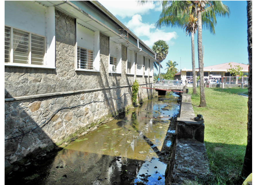
FIGURE 10 - St Fidele Library (V6083) abutting water drainage from Moosa River
