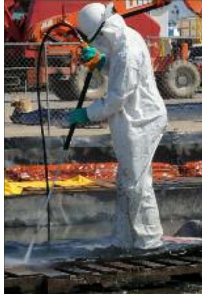
(Left) A worker power washes boom at the Deepwater Horizon Response Plaquemines Branch decontamination unit here, Aug. 19, 2010. As the workboats collect boom and deliver it to the decontamination area, personnel repair and clean it for use in a future response. (photo by PO3 Charly Hengen)
