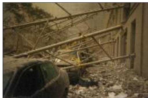
Sidewalk rubble near the WTC site on 9-11-2001
