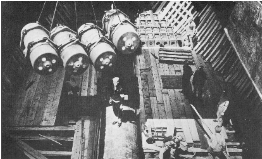
A member of an Explosives Loading Detail monitors the loading of high explosives and the work of carpenters as they construct the bombs’ wooden framework in the ship’s hold.
