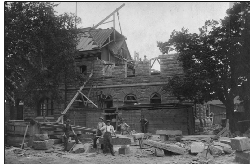
30 Russell Street East, 1914, rear addition
