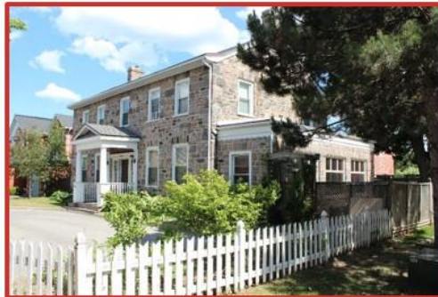
View of northwest corner (2016)
