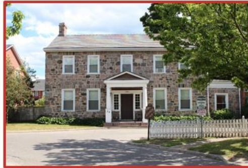
View of north façade (2016)
