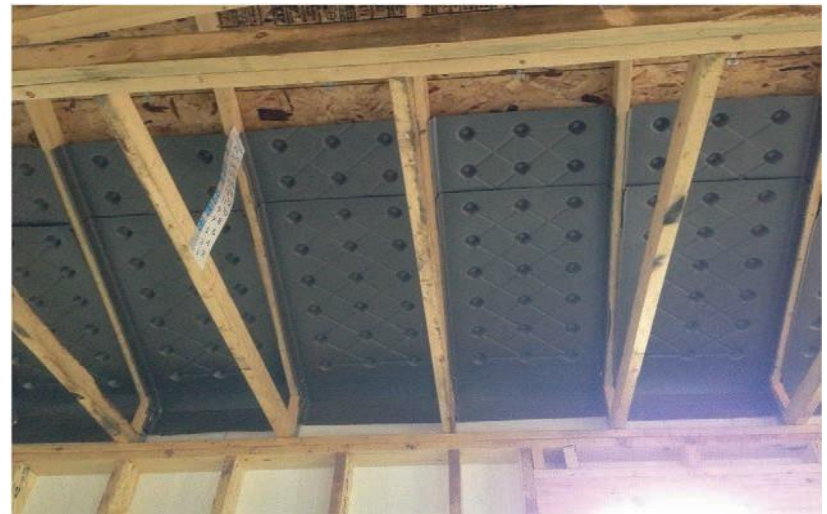
Baffles installed correctly
