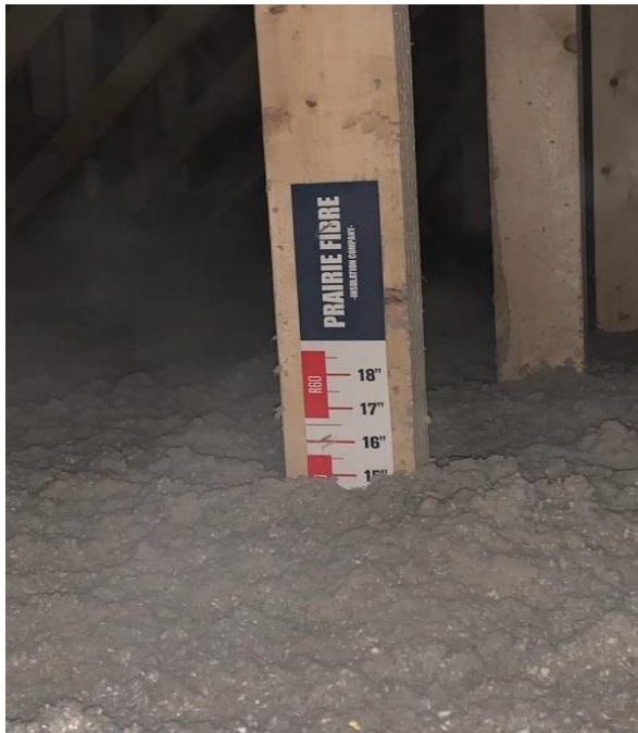
Properly installed Ruler matching Insulation Product
