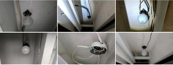
5. Main Basement Smoke Detector: Missing, Assessment: There should be a smoke detector in this room for safety purposes
