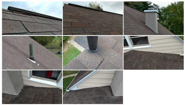
Plumbing Vent Flashing: Aluminum, Rubber
