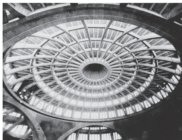
A dome of the Centennial Hall (1913) by Max Berg.
