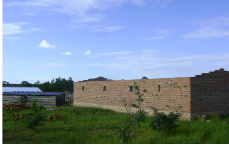
Storage shade to be roofed shortly
