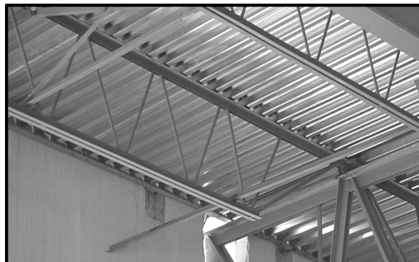
Photo 3: Lightweight Steel Construction
