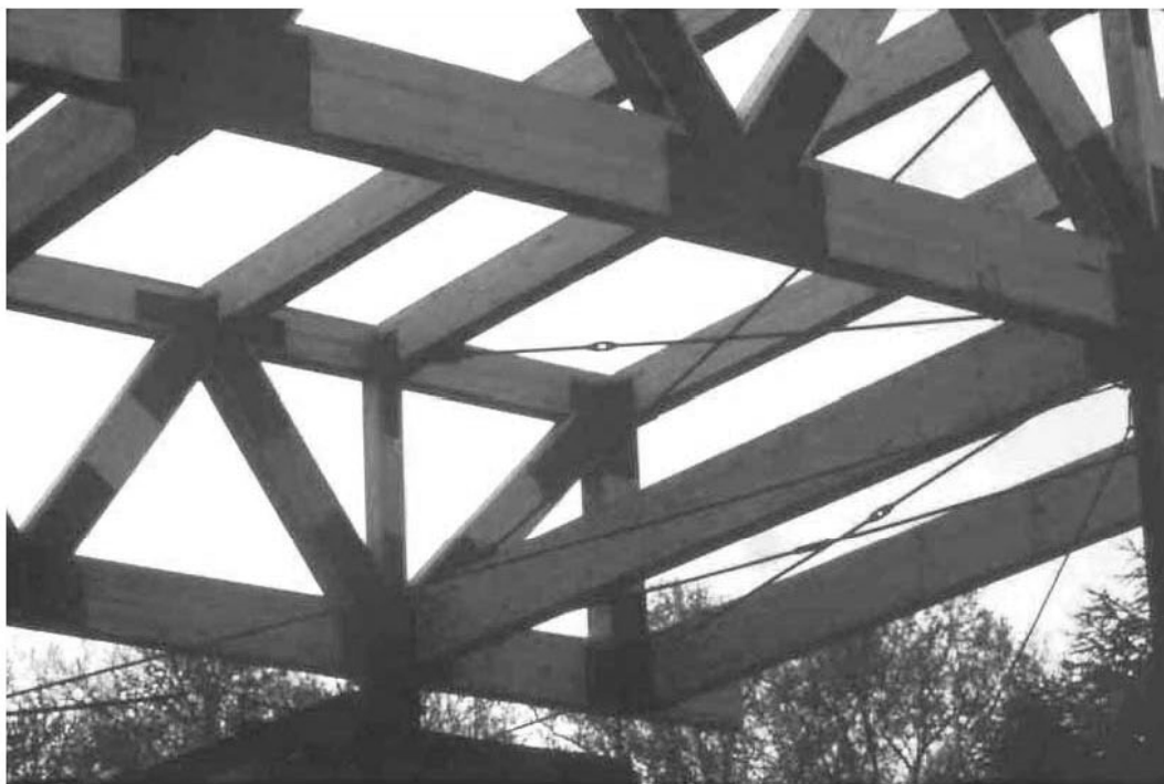
Figure E-1. Heavy timber truss with steel cable web members. (Photo courtesy of Francis Brannigan.)
