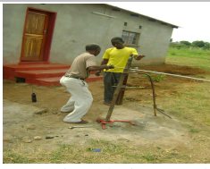
Water pipes being worked on
