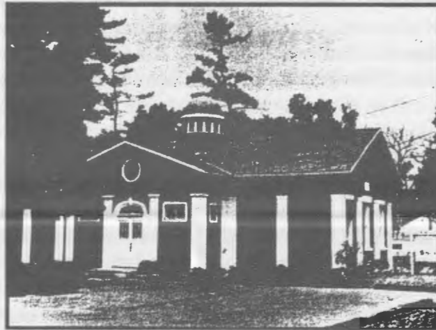
Cedar Hill School (1859). Home of the Town of Bethlehem Historical Association Museum. Route 144 (River Road) and Clapper Road.
