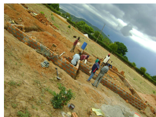
Sickbay/House being built & skills center foundations near main road
