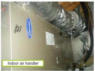
For your reference, heat pumps are used for heating and cooling of your home by transferring heat between two reservoirs. In the warmer months, the heat pump acts like an air conditioner, moving heat from inside your home to the outside. During winter months, heat from outdoors is transferred to the interior of your home. Amazingly, even a 32° Fahrenheit day still produces enough heat to warm a home via a heat pump.
