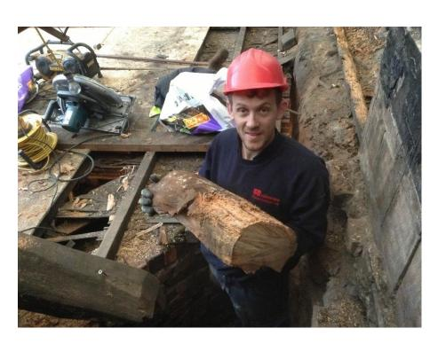
Matt the joiner of Robinson's Preservation is working on the roof timbers above the clergy vestry. The need for this urgent work is quite obvious when you see the rotten state of some of the timbers.
