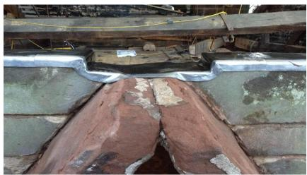
The great medieval walls of the clergy vestry need sealing, and lead is the only and best solution to the problem of damp in this situation. Now that the lead seal is in place, the heavy coping stones can be put back in place.
