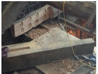
Robinsons ,the timber experts, are already hard at work rectifying the rotten beams, splicing new onto the old, as they have done so impressively in the Tower in Phase 5.
