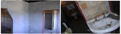
Plastering in progress & plumbing/wiring nearly done
