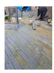
We ripped out an existing and rotten decking and replaced with brand new decking
