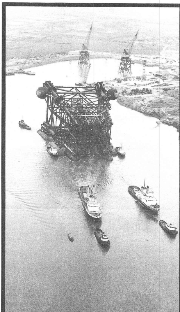
BP Photo ABOVE: BRITAIN'S first North Sea production platform "Graythorpe 1" being towed down Seaton Channel on its way to offshore oilfield. BELOW: A section of 36" pipeline is hoisted into position to be lowered into trench.
