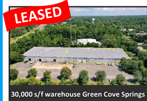
30,000 s/f warehouse Green Cove Springs
