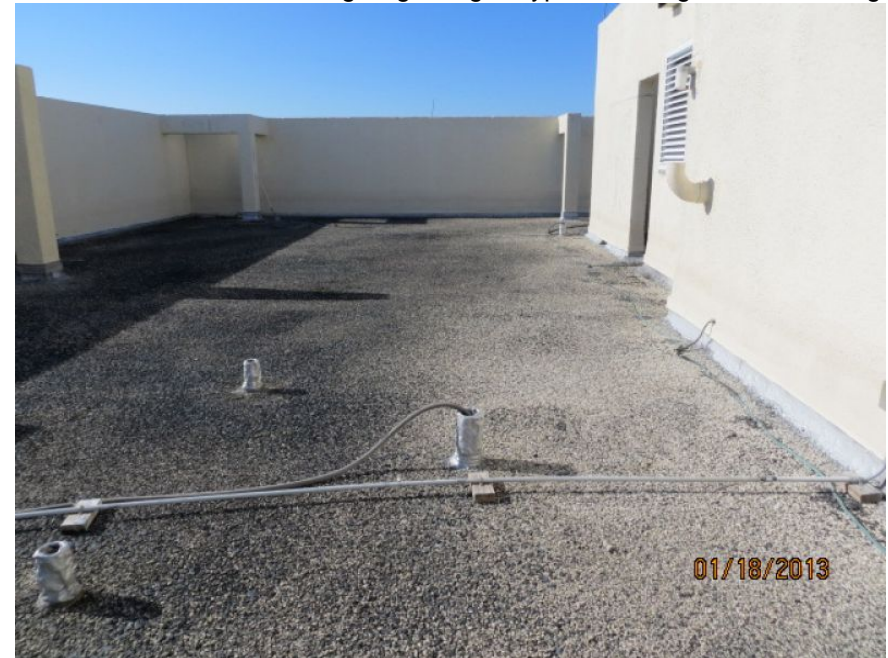
Built-Up Tar & Gravel Roof Covering
