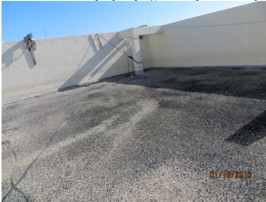
Built-Up Tar & Gravel Roof Covering
