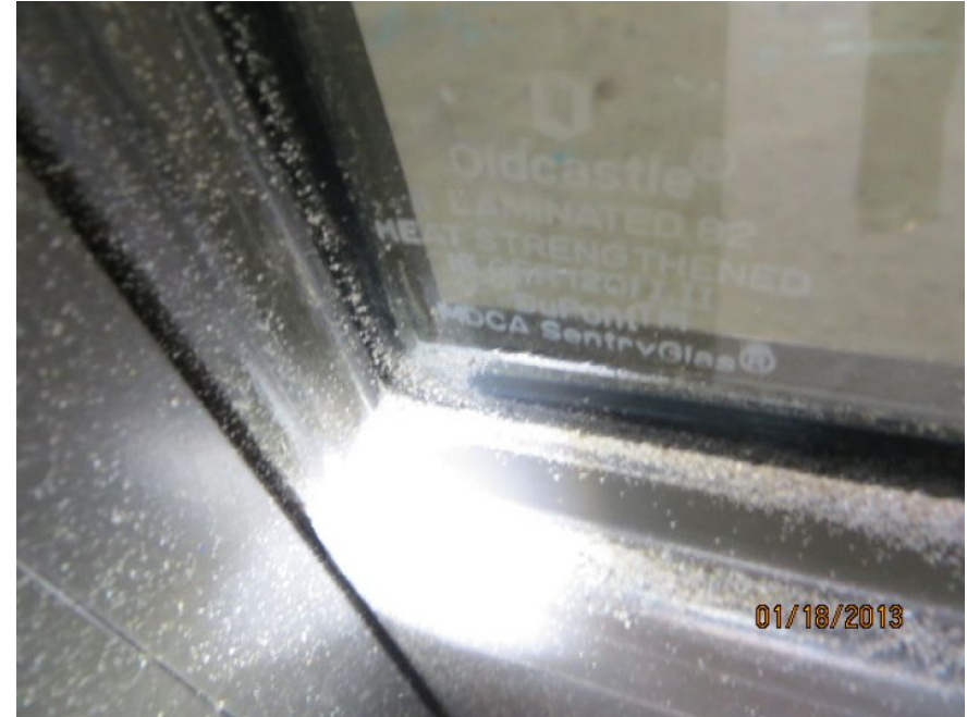
Impact Rated Glazed Door Etching/Engraving - Typical Throughout Entire Bldg
