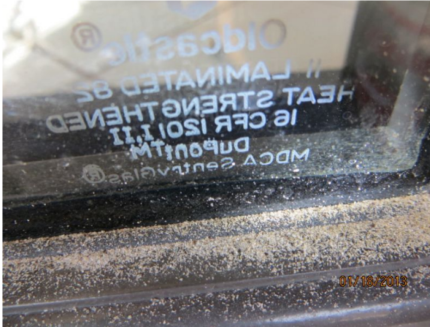
Impact Rated Window Etching/Engraving - Typical Throughout Entire Bldg
