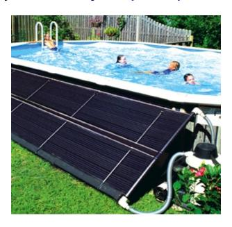
But before you decide, you'll need to answer some questions. First, will your solar panel system get enough sunlight during the day? The solar panels used for heating pools are simple passive collectors. They're typically made of plastic coils filled with water and sandwiched between sheets of shatter-resistant glass. As water collects in the coils, it gets heated by the sun then pumped into the pool.
