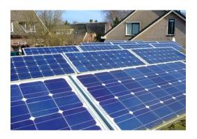
Solar photovoltaic cells create DC (direct current) electricity. Most typically, they use semi-conductor material (silicon) in the panel, which interacts with sunlight to create electricity. The electricity then can be used to power computers and appliances, or the entire house, if you build the system big enough. The
