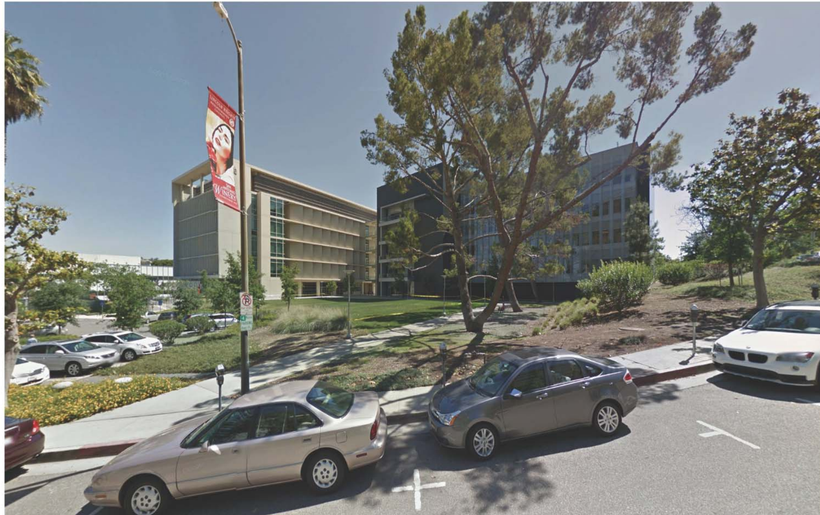
View of project site looking northeast from Eastlake Avenue
