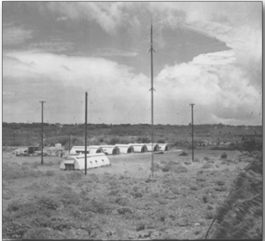
(Above) This was a typical USCG Loran-A station in the Southwest Pacific. Generally speaking, Loran-A had an average expected accuracy of 1 percent of the distance between the navigator and the stations according to the U.S. Coast Guard in 1949. (Photo courtesy Ken Laesser's Coast Guard History Page)
