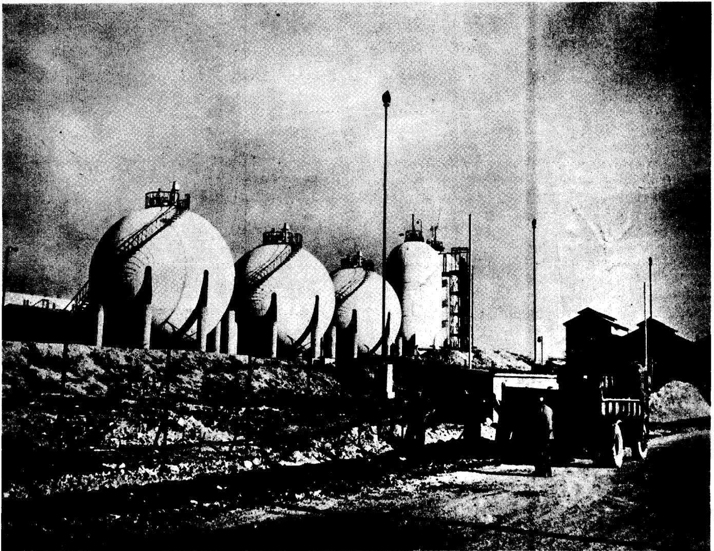
Wide World Photo Post-war butane gas storage tanks at the Shell Berre refinery, France. Though it has taken 15 years, Western Europe now leads the world in production.
